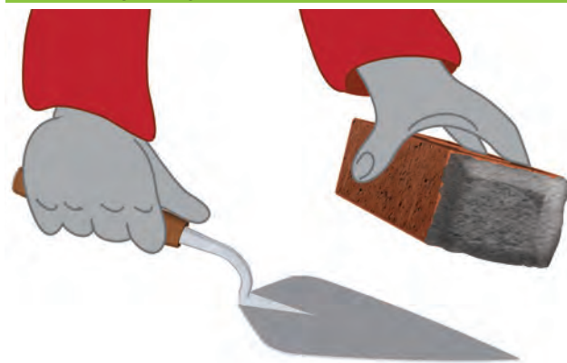
11.7 - Lifting enough mortar to butter a brick.
