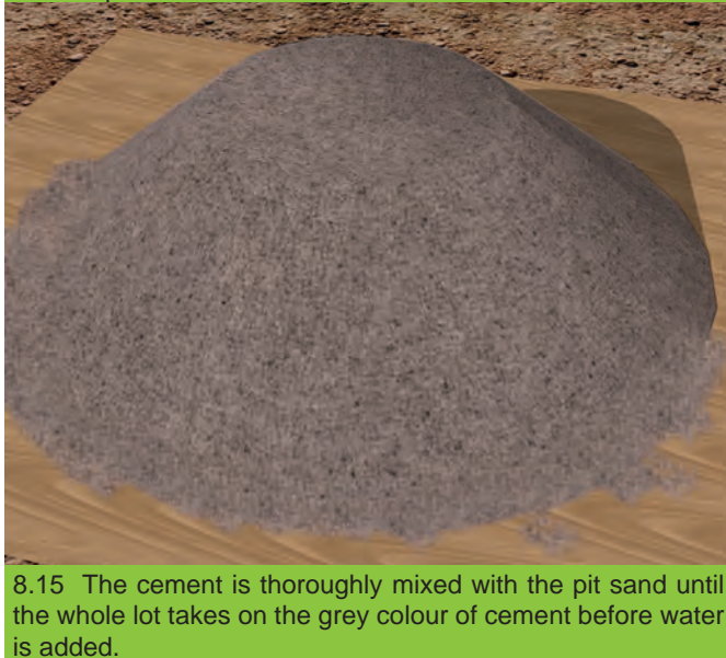
8.14 - Spread the cement over the mixture.
