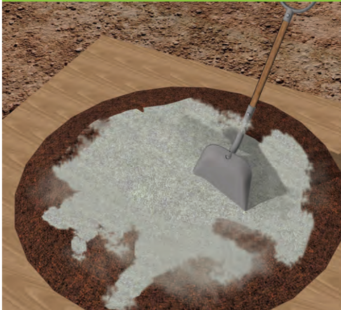
8.14 - Spread the cement over the mixture.
