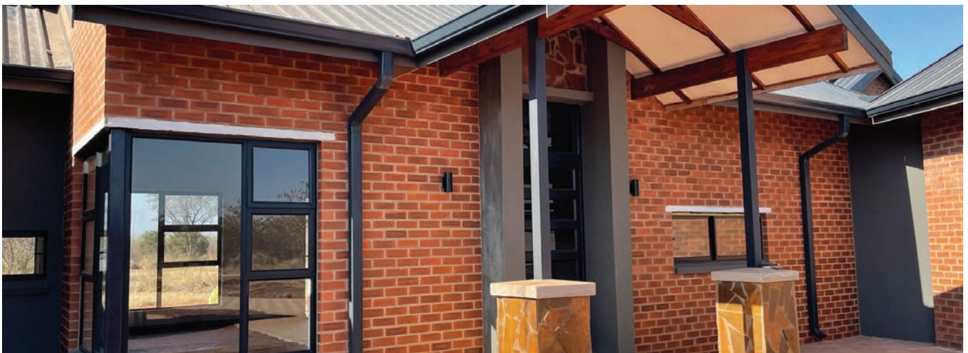
Home in Sondela Nature Reserve | Architect – 86 red BRICKS Architects
